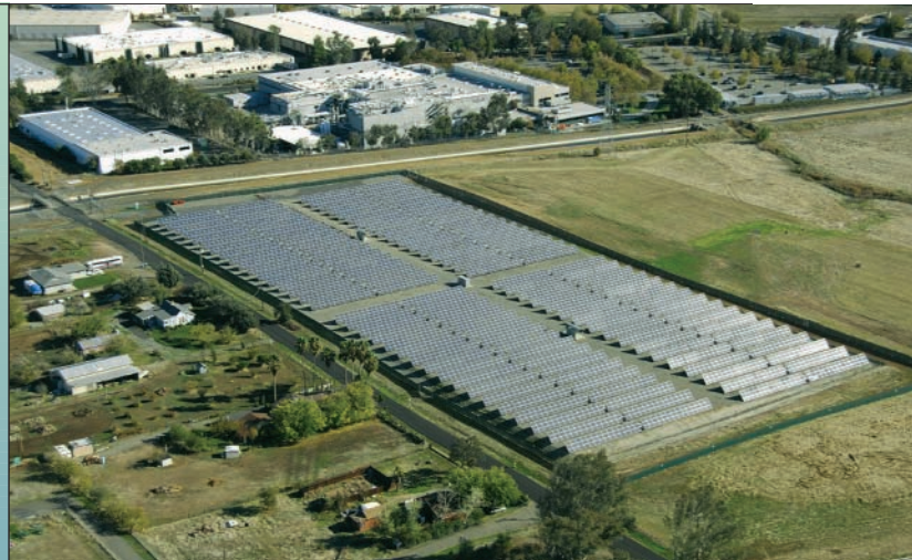
This 1.1-megawatt solar power system provides about one-third of the needed power for ALZA Corporation in Vacaville, CA when the sun is shining.
